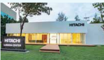
SHOWROOM AND OFFICE HITACHI LUMADA CENTER HITACHI ASIA (THAILAND) CO., LTD.
